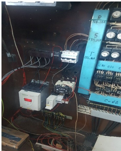
Fig. 8. New electrical panel
